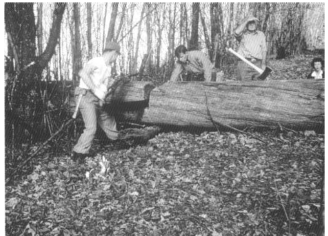
CMC Trail Work on the AT in 1958 Near Sam's Gap
