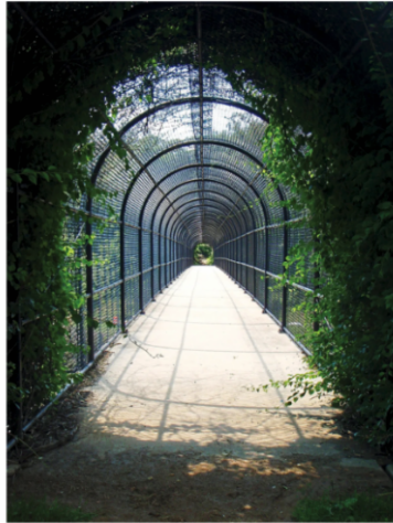
Over 140 tunnel, Maryland
